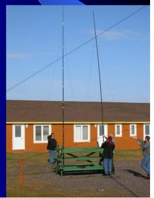
The mast was 38 ft tall and supported our 160M inverted V, the 30M/15M inverted V and the Yankee Clipper special 80M "C". The shorter mast had a 40M inverted V.
